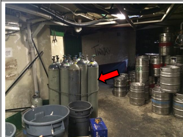
Photo 15: Correctly secured and stored gas cylinders
