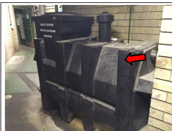
Photo 1: Grease trap in the lower level back of house area of the Robin Hood Hotel
