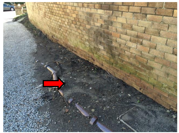
Photo 17: Exposed fill at 94 Carrington Road
