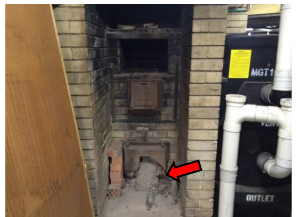
Photo 10: Disused incinerator adjacent to the grease trap on the lower level of the Robin Hood Hotel
