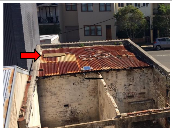
Photo 21: Discarded SMF insulation batts on the garage roof at 94 Carrington Road
