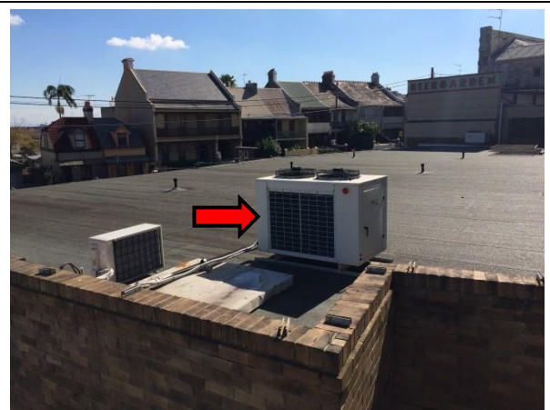
Photo 24: Air conditioning unit on the roof of the Robin Hood Hotel contains the refrigerant R22
