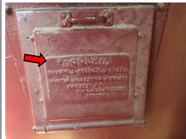
Photo 9: Chute for disused incinerator on the upper hotel level of the Robin Hood Hotel
