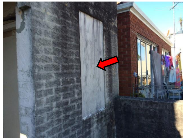
Photo 18: Asbestos containing fibre cement sheeting at 94 Carrington Road
