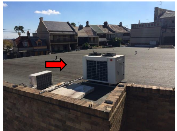
Photo 19: Asbestos containing bituminous membrane on the roof of the RHH
