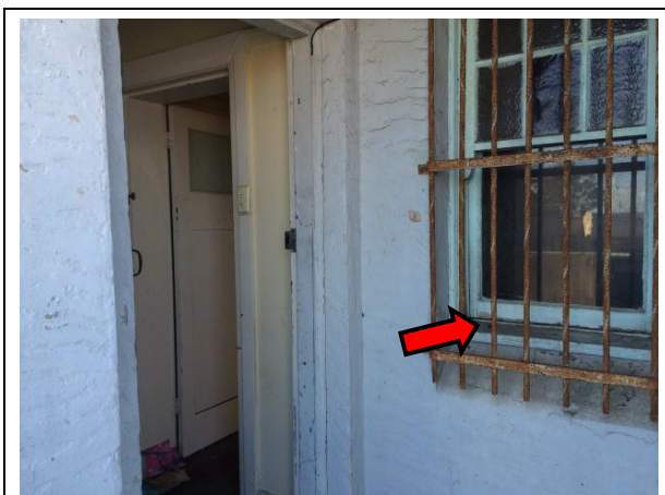
Photo 22: Lead based paint on the exterior window frames of the apartments at 94 Carrington Road
