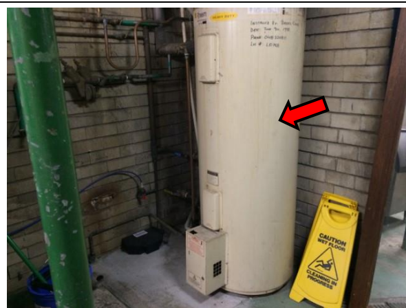
Photo 20: SMF insulation within hot water heater at the Robin Hood Hotel
